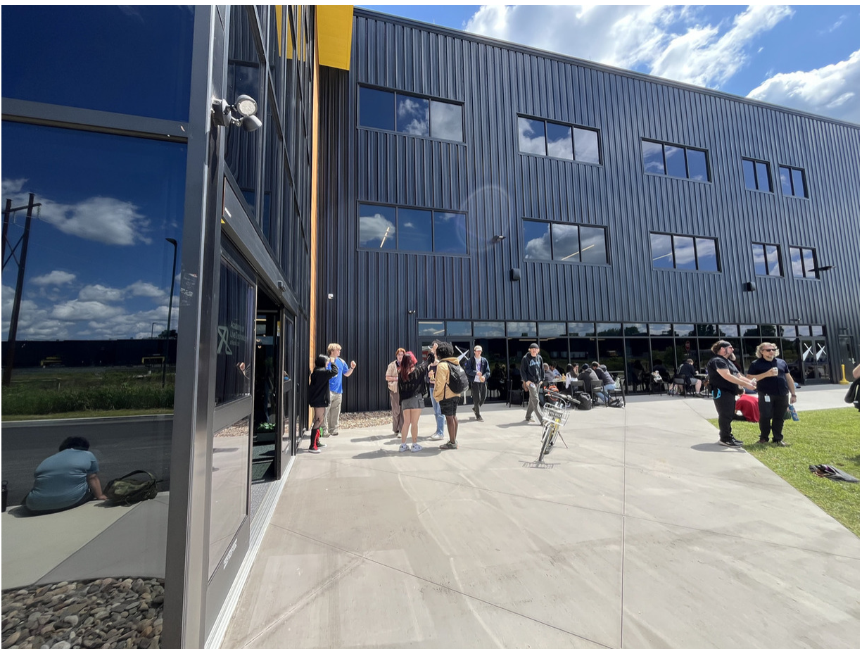
Students and faculty visit outside the new ALT facility that opened last month at Rock Litz.
